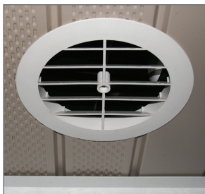
EZ Soffit Vent installed
