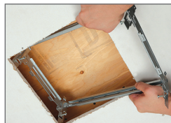
Insert single-hinged Flex-Z Fast® installation bracket
