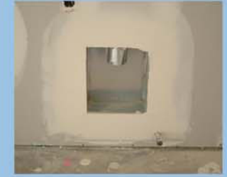
shop made dryer vent boxes
