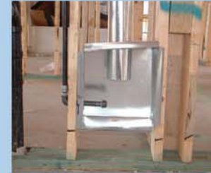
shop made dryer vent boxes
